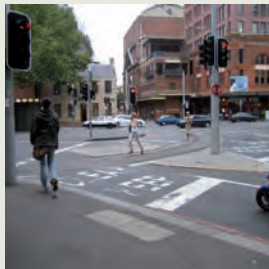
The crossing between Hay Street and Belmore Park is broken into many pieces.
