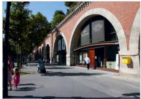
Paris, Promenade Plantée / Viaduc des Arts: abandoned elevated train line is transformed into an attractive walk with ateliers inside and a new park on top (1990)
