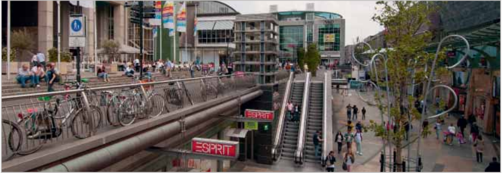
Shopping centre Beurstraverse in Rotterdam
